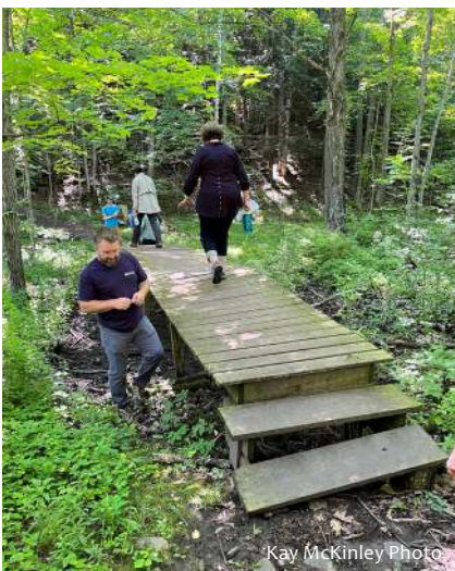
A new trail bridge will be built at Bay Shore Blufflands.
